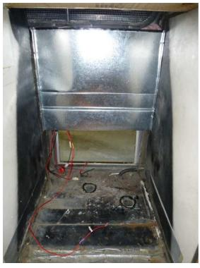
Seemed odd, but it makes some sense. He has since changed to blocking 2/3 of the bottom vent and is reporting that the fridge is rock steady when driving.
